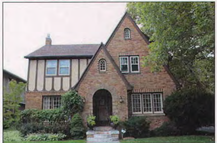
1704 Herbert Ave. Built 1927 by Philip Biesinger Multi-color brick, half-timbering English Tudor Jacobethan Revival
