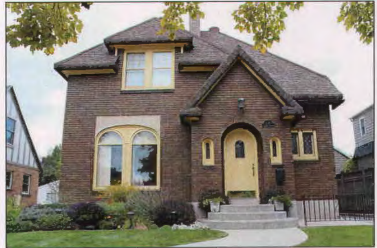
1757 Herbert Ave. Built 1928 by Philip Biesinger Regular brick, rolled roof English Cottage French Norman
