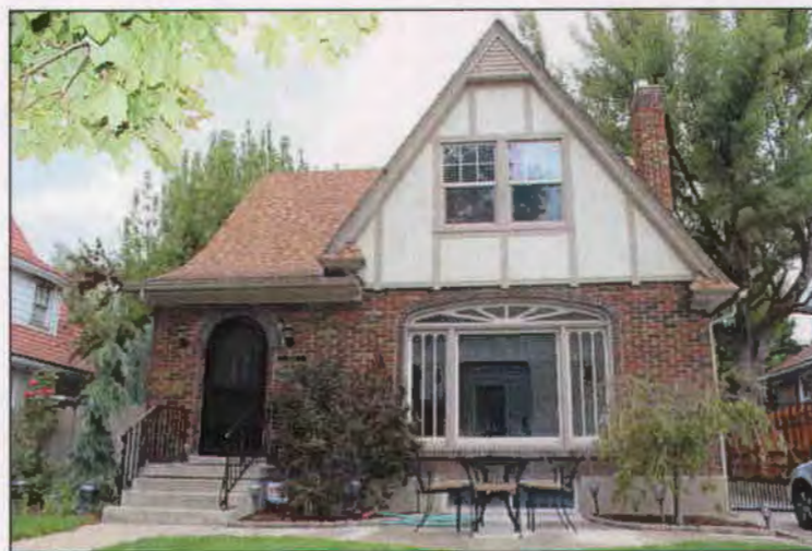
1733 Herbert Ave. Built 1927 by Philip Biesinger Regular brick, siding added later English Cottage
