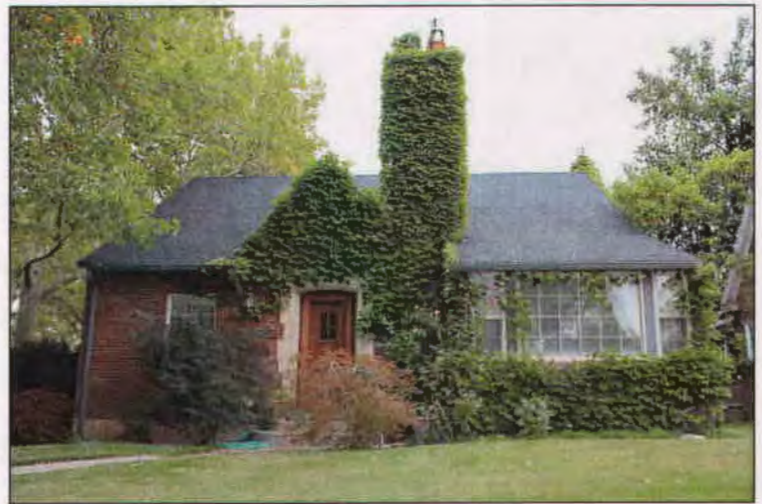
1703 Herbert Ave. Built 1936 by Capitol Building Striated brick English Cottage Jacobethan Revival
